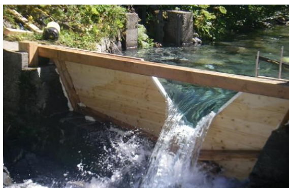
Figure 8 Example of a V-notch weir with wood plate ( http://www.dransenergie.ch/ )
